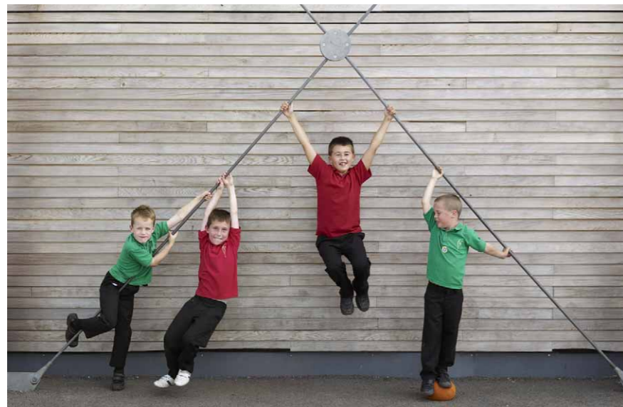
Left: Kingsmead is intended to allow the schoolchildren to appreciate the benefits of lightweight and ecological building. The construction of the school was therefore left openly visible and would even be usable for gymnastics.
